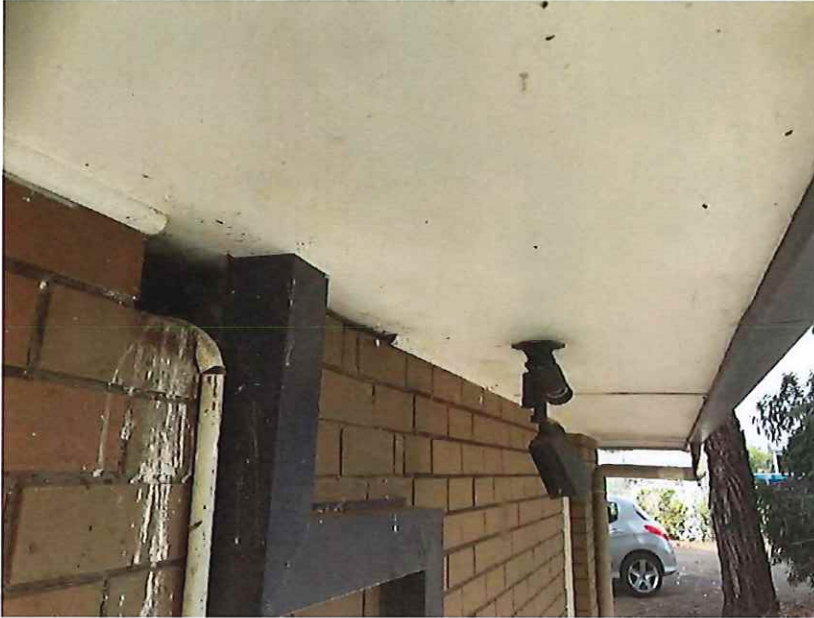
Photo 1-External, Eaves – asbestos-containing white painted fibro-cement
