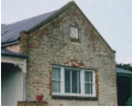
laurence park homestead buchter road batesford front window detail publication
