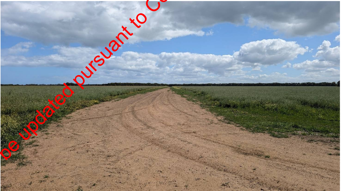
Image 6: The existing runway to be used for the farm track.
